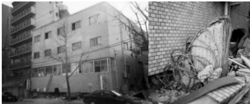
Photo 1 Damaged four-story pilotis building
