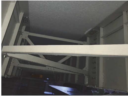
(c) Lateral bracing
