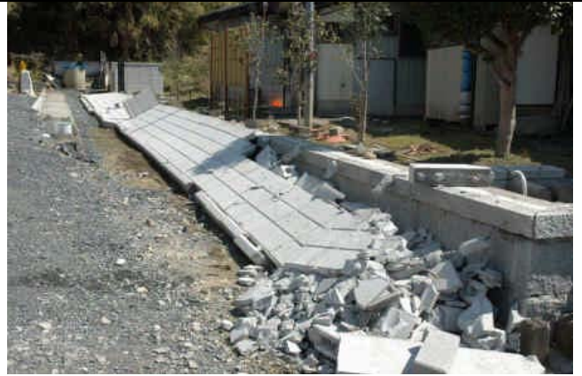
Photo 4: Fall of a guardian dog statue and also concrete block walls along a lot
