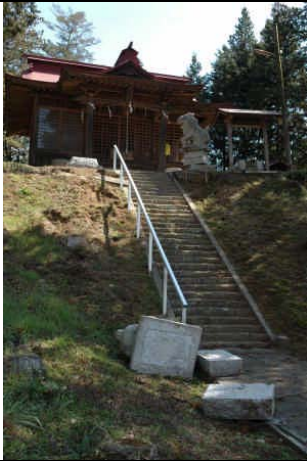
Photo 4: Fall of a guardian dog statue and also concrete block walls along a lot
