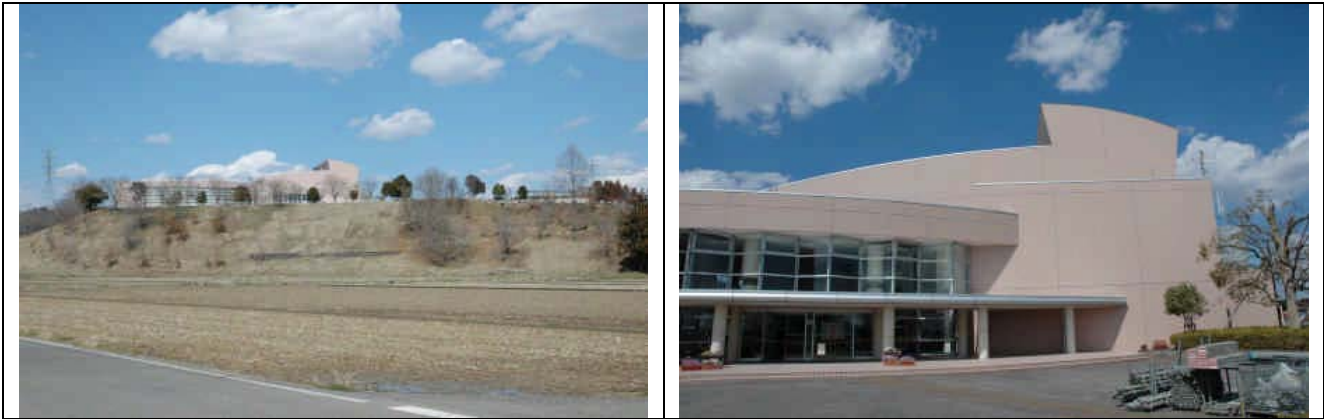
Photo 15: Overall view of the Municipal Exchange Center Building
