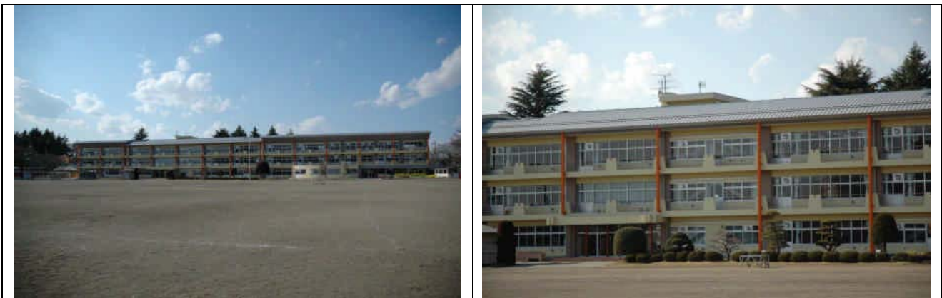
Photo 18: Overall view of Godai Elementary School
