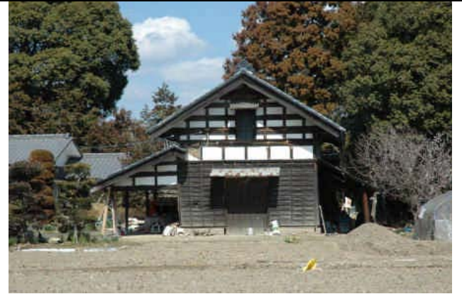
Photo 6: Damage on roof tiles and a tilted traditional barn
