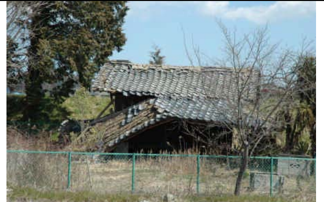
Photo 5: Collapse of timber barns
