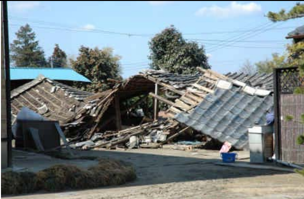
Photo 5: Collapse of timber barns
