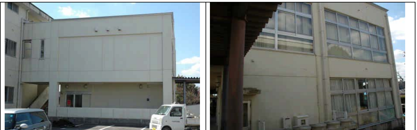
Photo 12: Overall view of a visual and audio education building.
