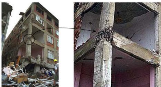
Figure 2. Joint panel damage caused by earthquake (Guner, 2016)
