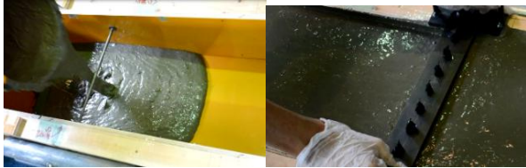
Figure 3. Placing and moving a comb device
