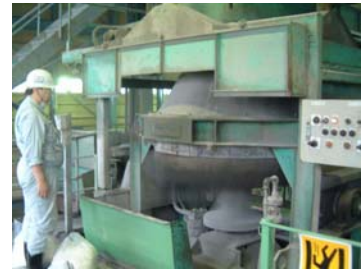
Fig.2 Omni mixer in actual plant
