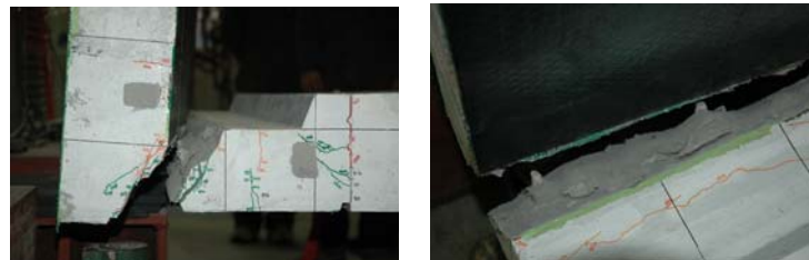
Figure 6 Final collapse section in PCD-3
