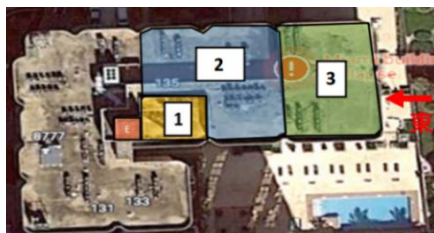
Fig. 1 Plane aerial view of Champlain Towers South (2)
