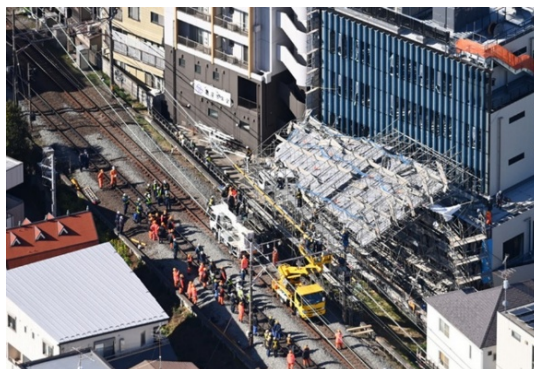
Figure 1. Accidental collapse of scaffoldings due to strong winds occurred in Tokyo on March 2 nd , 2021[1].
