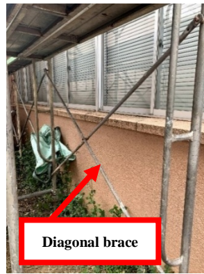
Figure 4. Diagonal braces.
