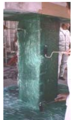
Photo 2: Surface curing
